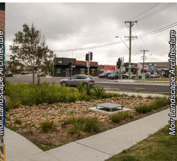
WSUD system adjacent to roadway, Glebe Road, Newcastle
