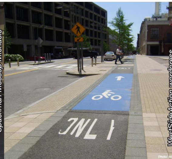
Raised pedestrian crossing over vehicular driveway access
