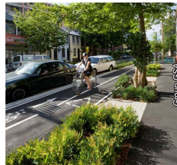
Median barrier planting with street trees as a separating barrier, Bourke Street, Sydney
