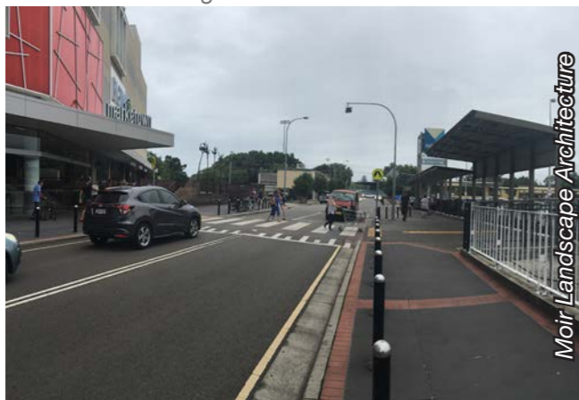
Pedestrian crossing at Cottage Creek
