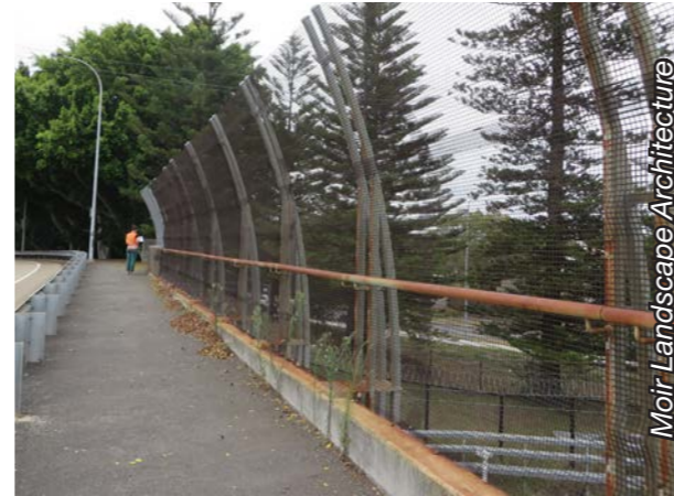
Rail bridge overpass, Hunter Street
