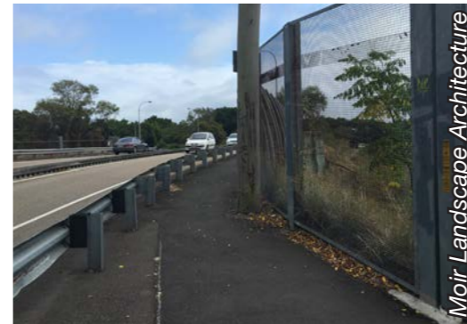
Railway bridge, Hunter Street
