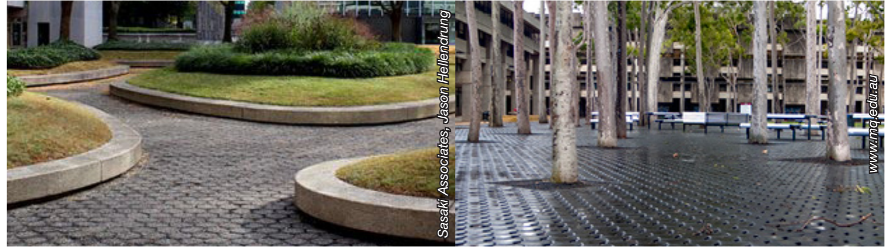
Proposed raised grassed planters with seating walls, Constitution Plaza, Hartford, CT, United States
